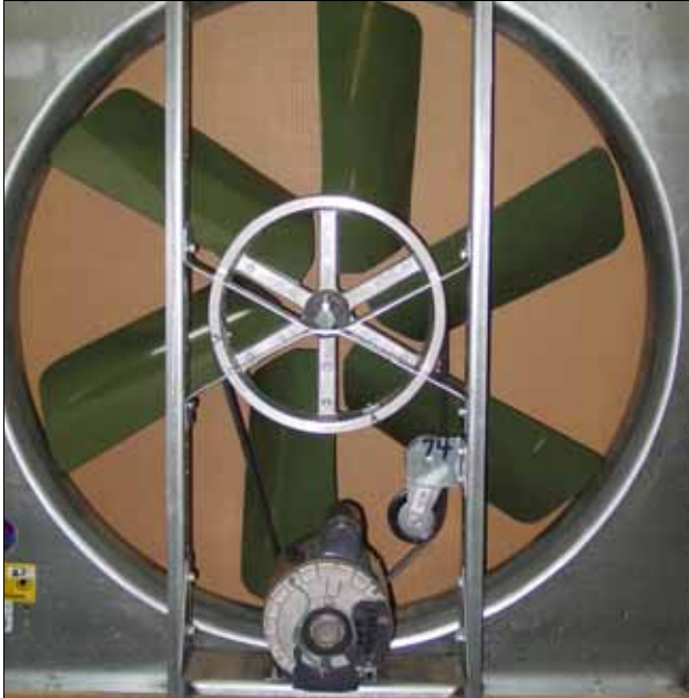
NCFA36 with motor mounted at the bottom of the fan
